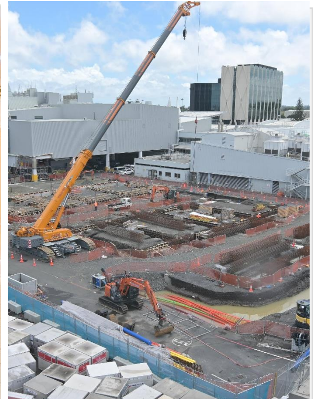
Foundation work on the Eastern Bag Hall
