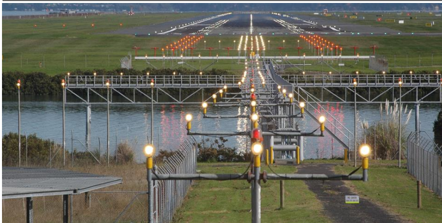
Purchase of Airways' airfield lighting
