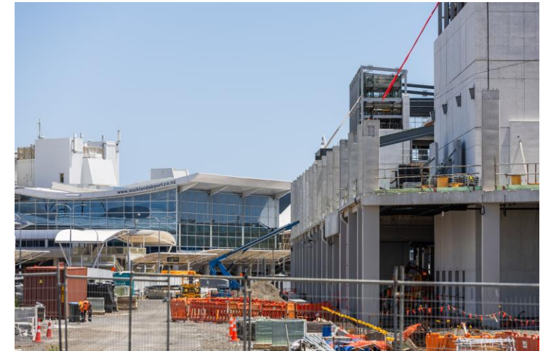
Construction of the Transport Hub
