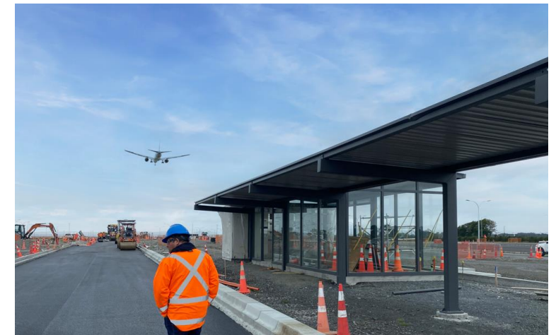
Construction of Park & Ride South
