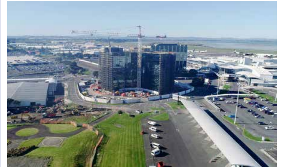
Te Arikiniui Pullman Hotel – under construction
