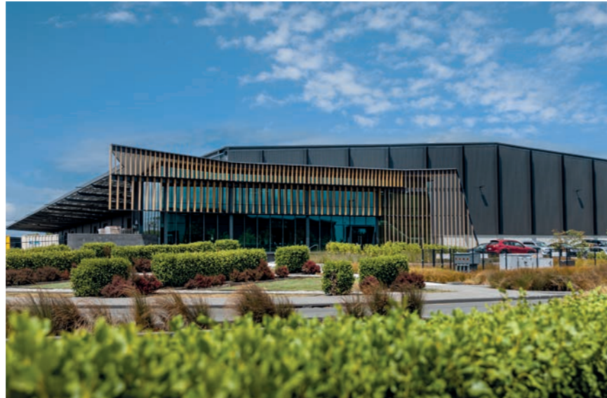
The EBOS Group development at The Landing Business Park
