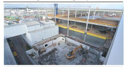
Multi-year programme of enabling works to relocate infrastructure and prepare the site for the construction of a new domestic jet pier and headhouse integrated into the existing international terminal building (refer Domestic Processor 2nd column)
