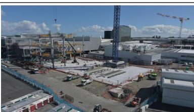
Multi-year programme of works to enable the delivery of a new domestic jet pier and headhouse integrated into the existing international terminal building.
