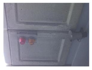
evacuating onto the ramp or an apron Emergency Assembly Point. These are installed near entrances to the ITB on the apron. Red flashing lights indicate that an alarm is taking place within the building and not to enter this part of the building. Amber flashing lights indicate that an alarm is sounding in an adjacent building zone and you should enter the building with caution.
