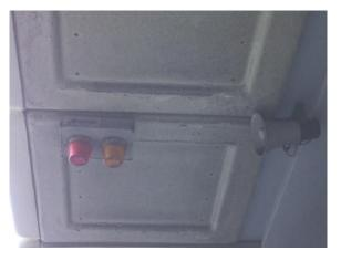
evacuating onto the ramp or an apron assembly area. These are installed near entrances to the ITB on the apron. Red flashing lights indicate that an alarm is taking place within the building and not to enter this part of the building. Amber flashing lights indicate that an alarm is sounding in an adjacent building Zone and you should enter the building with caution.
