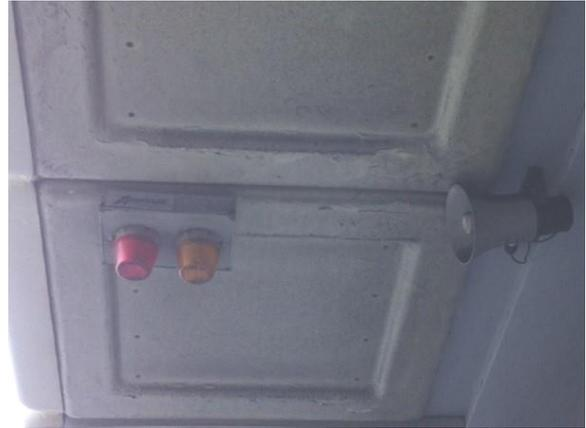
D5.4 A red strobe on the building will activate when people in an adjacent zone within the building may be evacuating onto the ramp or an apron Emergency Assembly Point. These are installed near entrances to the ITB on the apron. Red flashing lights indicate that an alarm is taking place within the building and not to enter this part of the building. Amber flashing lights indicate that an alarm is sounding in an adjacent building zone and you should enter the building with caution.
